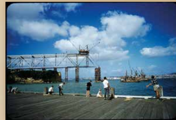
Auckland Harbour Bridge under construction. It was completed in 1959. Auckland Libraries, 654-26 (Geoff Fairfield).
