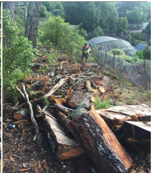
Photo No.2: Result of 'dismantle and leave on site'
