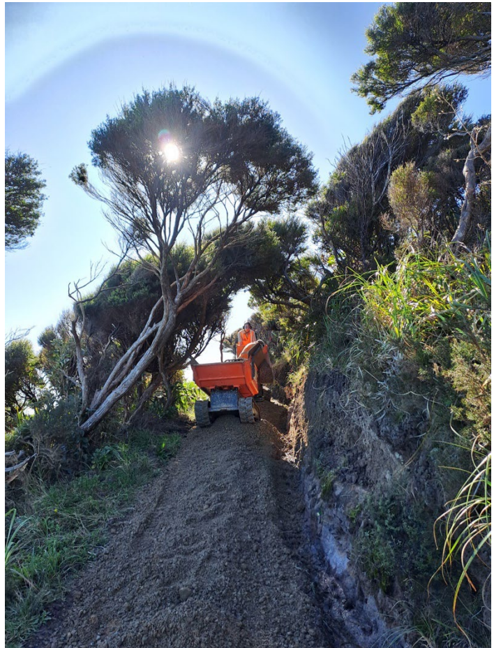
Work underway at Mercer Bay Loop track.
