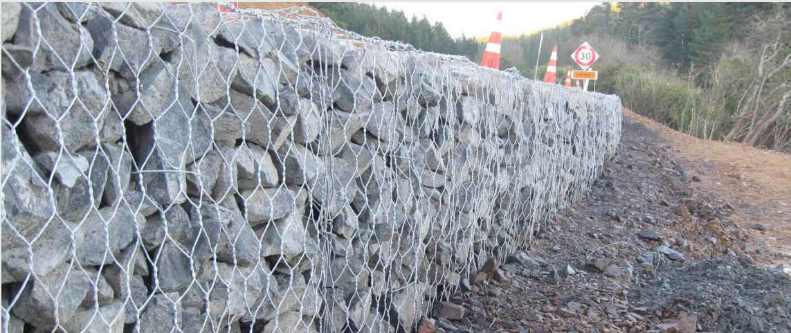
Gabion (rock) wall example
