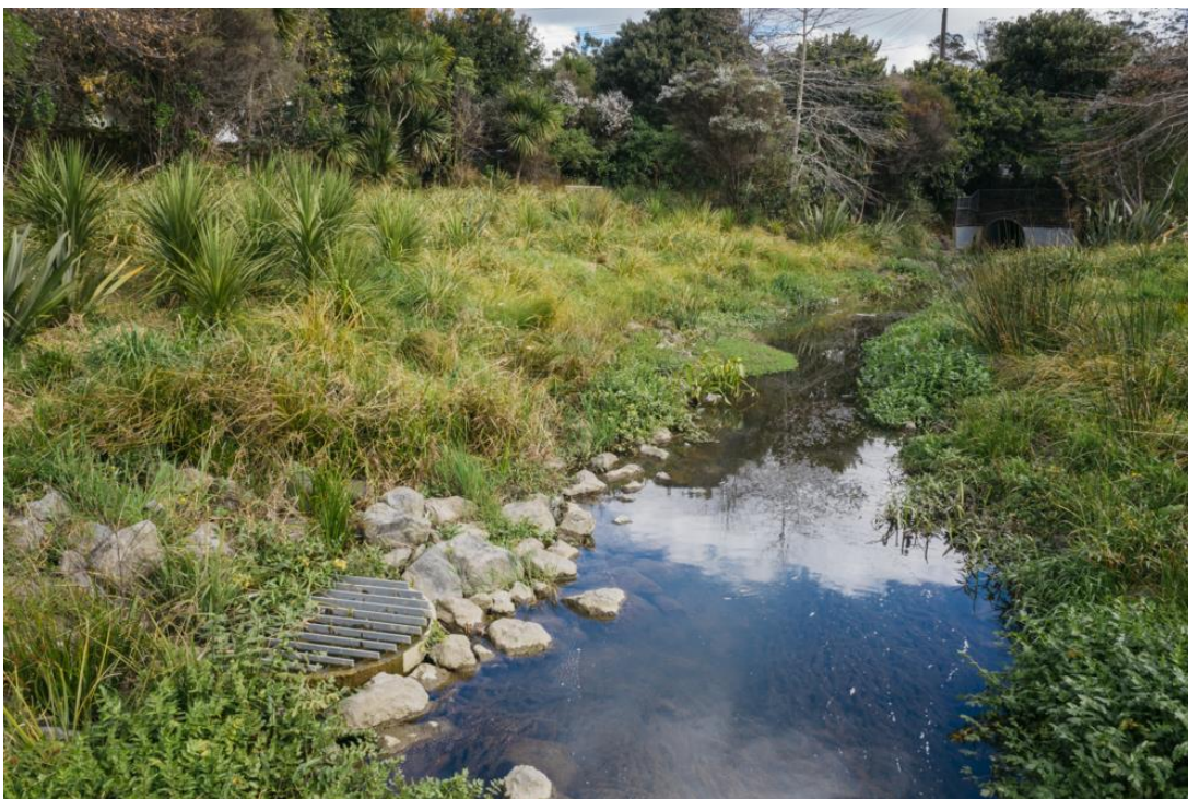
D'Oyly Reserve Stormwater Project, Stanmore Bay
