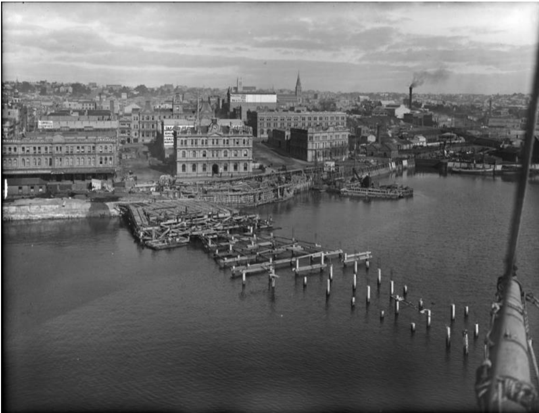
Figure 9. Auckland waterfront in 1907, showing construction of the (existing) Ferry Terminal Pier 2. The Sturdee St Graving Dock (far right of photo) is still present at this time (Sir George Grey Special Collections, Auckland Libraries, 1-W1427)
