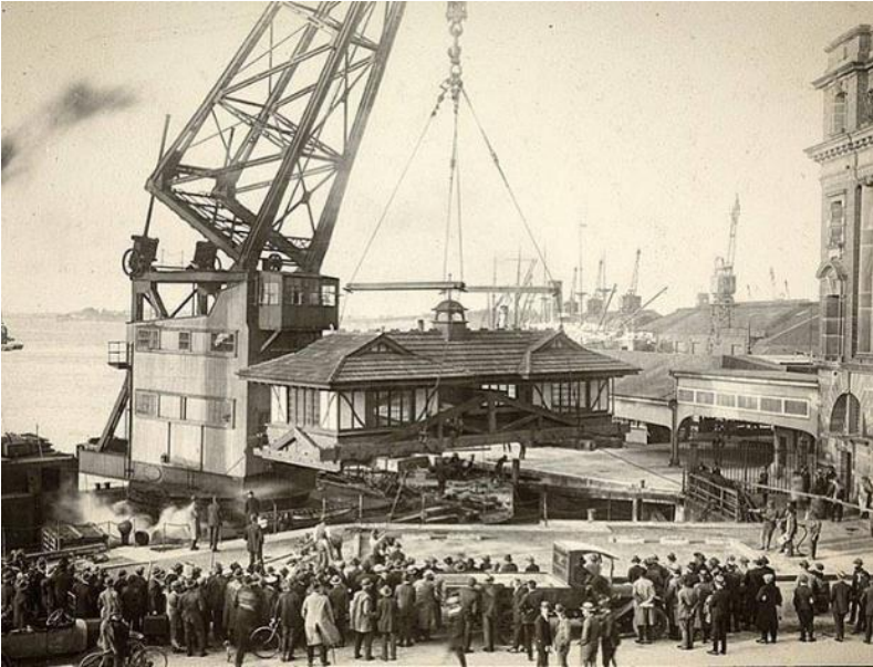
Figure 18. 1922 image showing the relocation of the Eastern Ferry Shelter to its current location. "In order not to damage the shed, which has a tiled roof, the foundation was cut away, and a cradle built of 12 by 12 hardwood timber was placed under each end of the building. To these cradles a bridle was attached ... According to the gauge on the crane the shed weighed 25 tons." (NZ Herald 2 November 1922)
