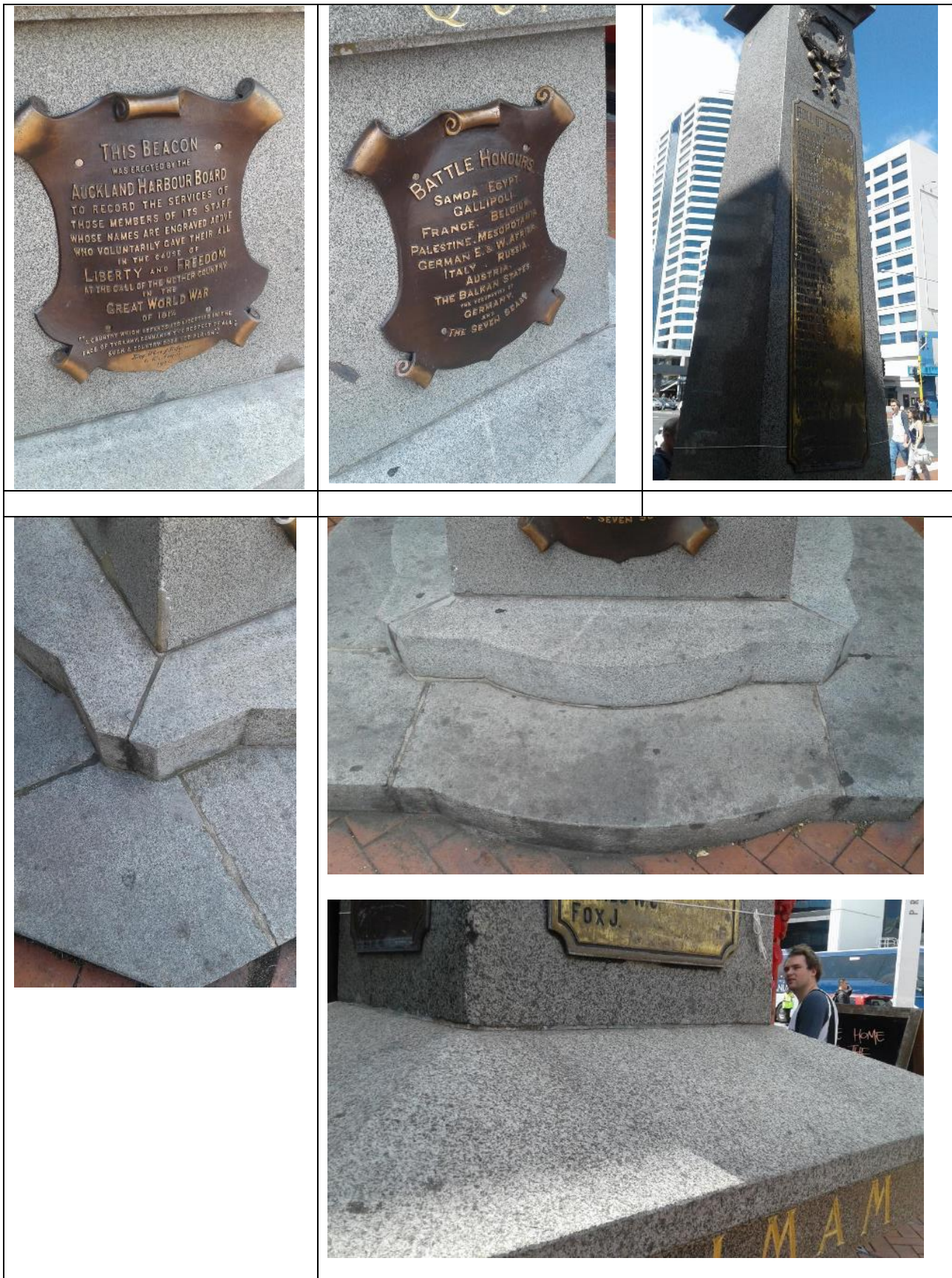
Figure 34. The Beacon, showing construction and details
