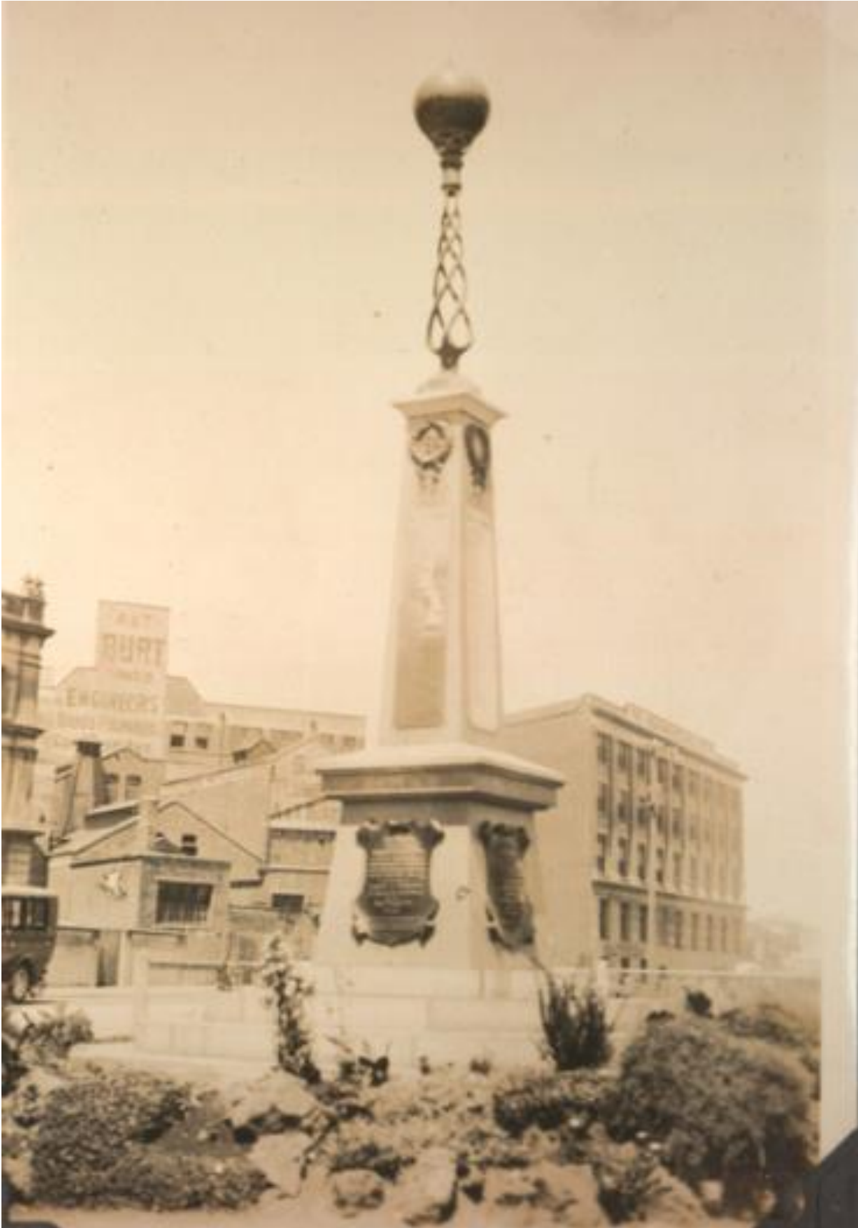
Figure 11. Undated photograph, showing original features, as well as rocks and planting around the base of The Beacon (New Zealand Maritime Museum, Foss Tackaberry: Undated)
