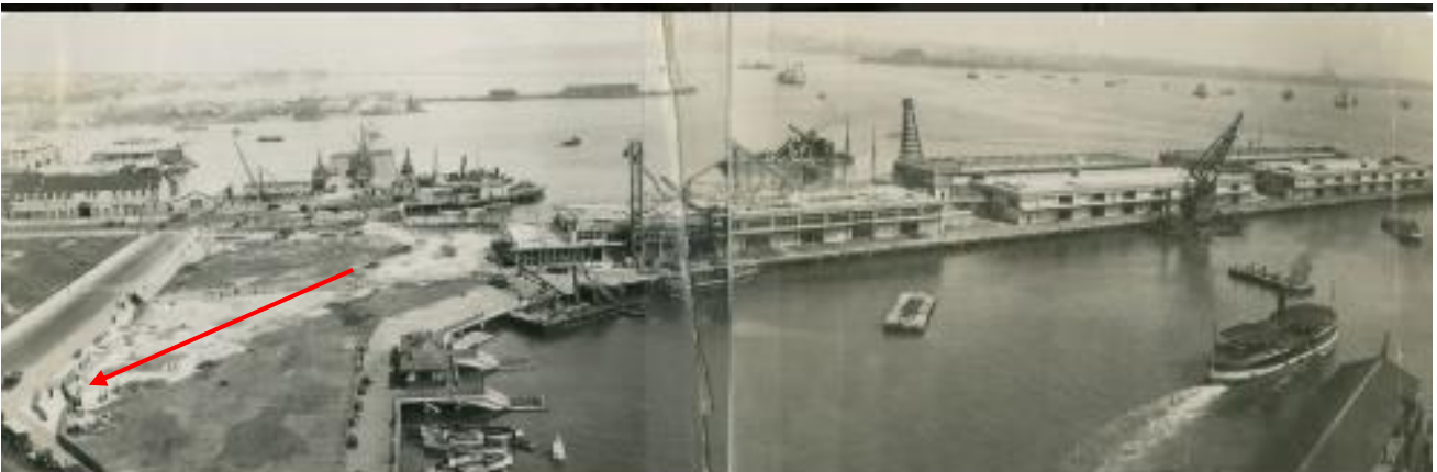
Figure 17. Princes Wharf from Ferry tower, 8 February 1924, showing reclamations between The Beacon and new waterfront. Note the seawall has been extended westwards to meet the new Princes Wharf (Auckland Harbour Board photo album no. 10, Voyager New Zealand Maritime Museum). The red arrow shows the location of The Beacon.
