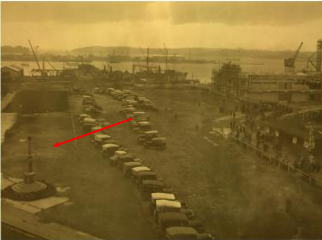
Figure 20. Cars parked on recently completed reclamation south of Princes Wharf, 12 May 1924. Picture shows The Beacon (left, location arrowed), now on south side of Quay Street, with Princes Wharf under construction (right) (Auckland Harbour Board photo album no. 10, Voyager New Zealand Maritime Museum)
