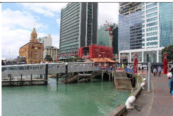
General view of Quay Street and Ferry Basin from Princes Wharf looking SE
