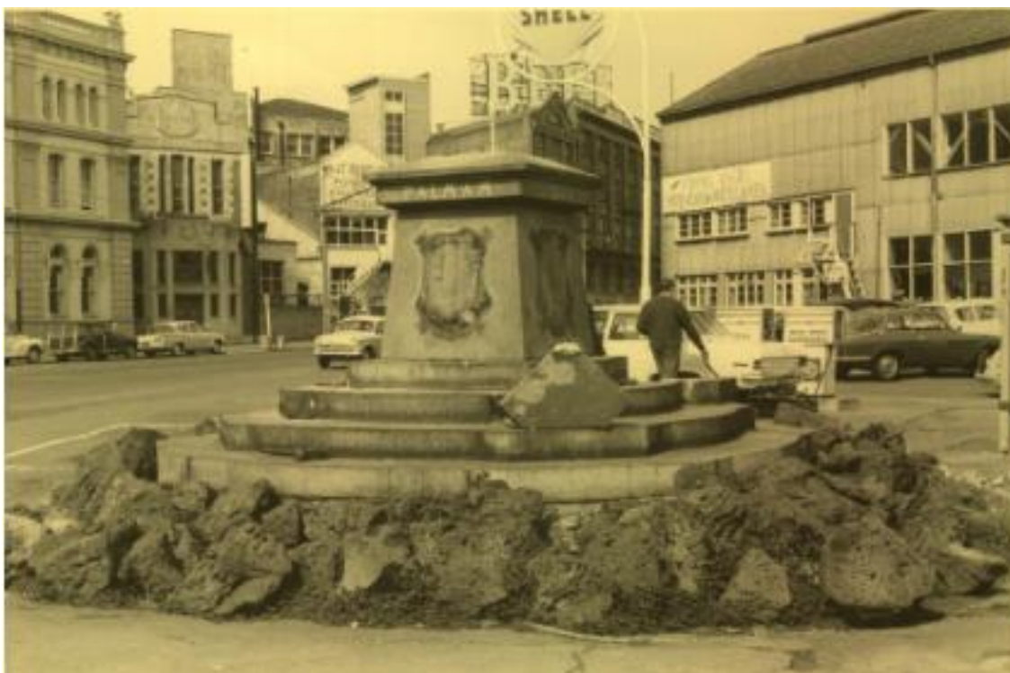
Figure 23. Base of obelisk, corner Sturdee and Quay Streets, showing its construction with no planting in c.1970 (Auckland Harbour Board collection, Voyager New Zealand Maritime Museum)
